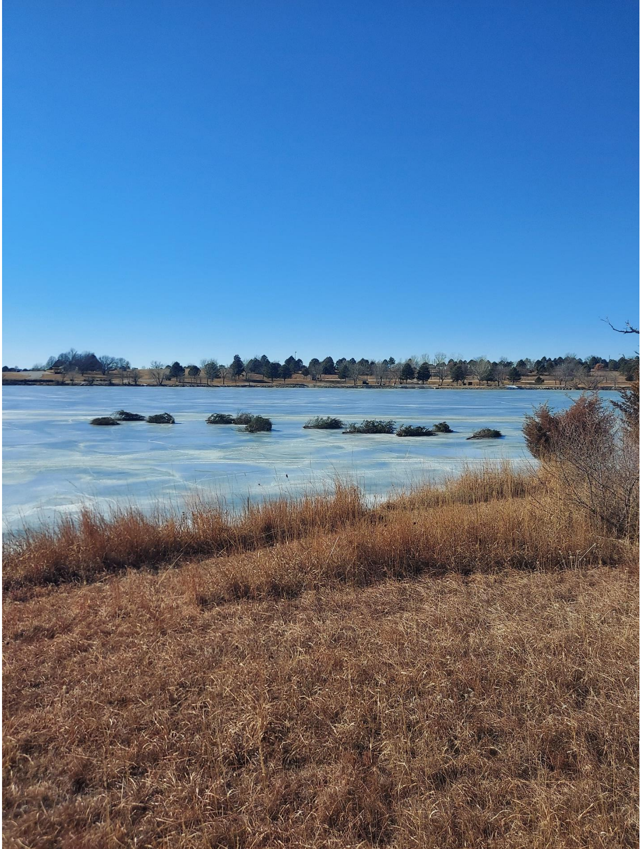
Cedar tree piles placed on top of the ice with blocks attached
