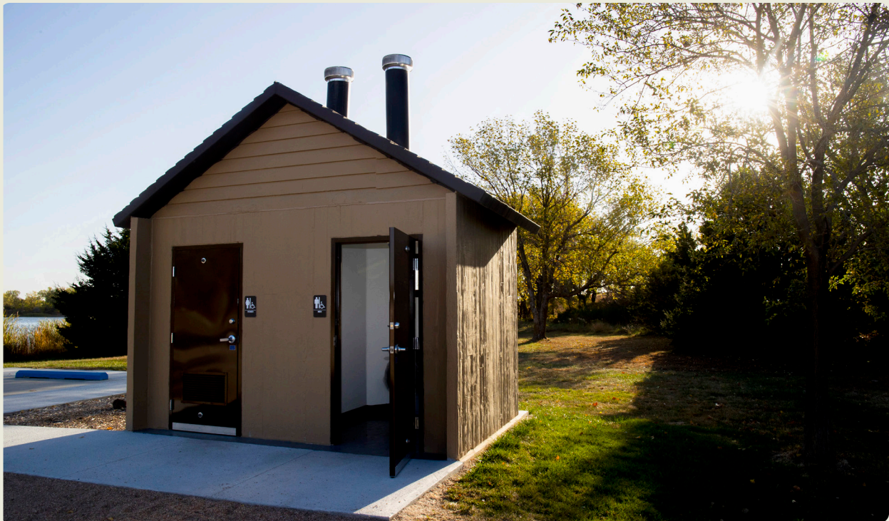
Mormon Island State Recreation Area received a new vault toilet using Capital Maintenance Fund dollars.
