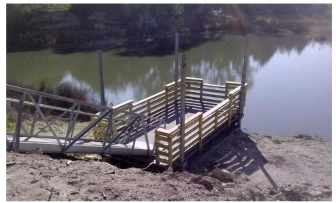
Left: New fishing pier installed at the trail 2 area. This picture is taken a t a very low lake level and is a floating pier at normal operating elevations.
