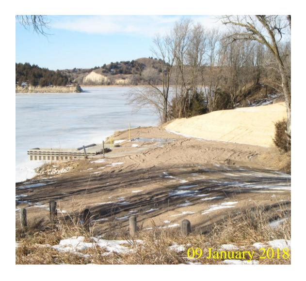
During 2017, construction occurred at the WMA boat ramp area. This improvement project was done to permanently replace the floating dock, improve drainage, allow ADA access and enhance bank angling opportunity. Although this project is not 100% complete at the end of 2017, it is near. This was a joint project between NGPC and CNPPID. Access CNPPID's News Release for more details.
